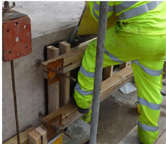
applied in sections generally up to 200 mm thick although greater thicknesses may be achievable dependent on the configuration of the repair location and the volume of exposed reinforcing steel. Consult the local Fosroc office for further information.
