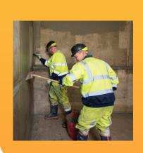
When mixed with clean water and applied correctly, **Tanking Slurry** forms a permanent waterproof coating to the concrete and masonry and is easily applied by brush, roller or spray.
